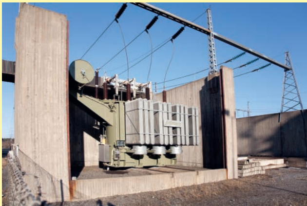
▲ Figure 4.5.34 Step-up transformers at a power station
