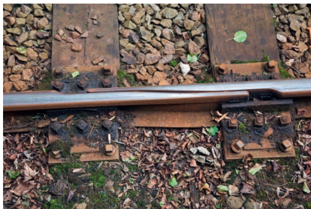
▲ Figure 2.2.4a Tapered overlap of rails
