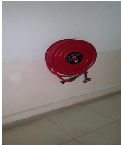
Plate xvi: showing the fire control hose reel located at the entrance of the building. Source: Authors field work
