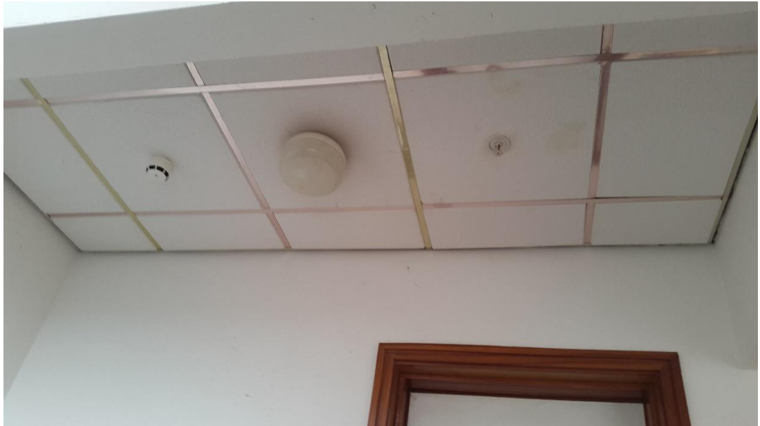
Plate xiii: showing the fire sprinkler and smoke detector. Source: Field Survey
