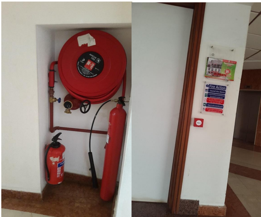
Plate xii: showing the fire hose, extinguisher and Alarm button
